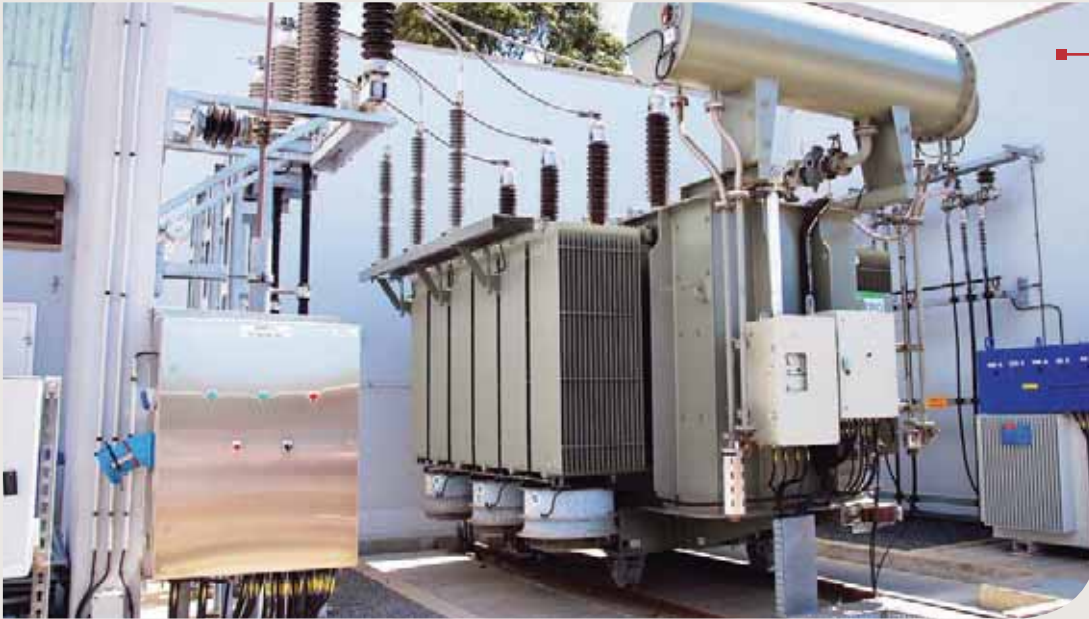
MAMOUDZOU, THE CAPITAL OF MAYOTTE, WAS SUPPLIED FOR THE FIRST TIME AT THE END OF 2014 WITH THE 90,000V HIGH-VOLTAGE CABLE WHICH CONNECTS THE LONGONI THERMAL PLANTS TO THE KAWENI TRANSFORMERS.
