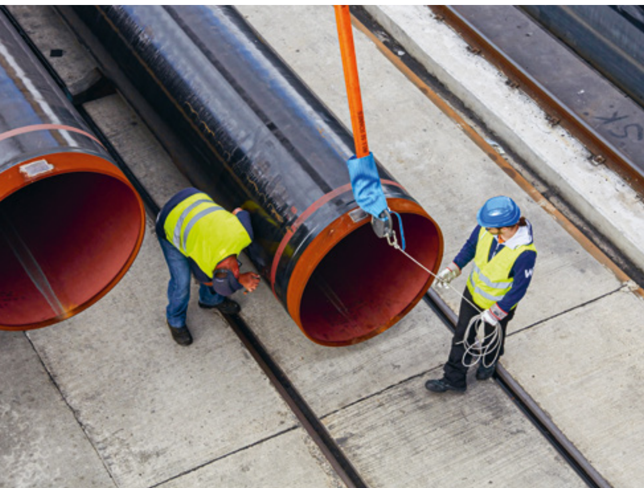
Unloading pipes transported by barge in the port of Frouard. © GRTGaz
