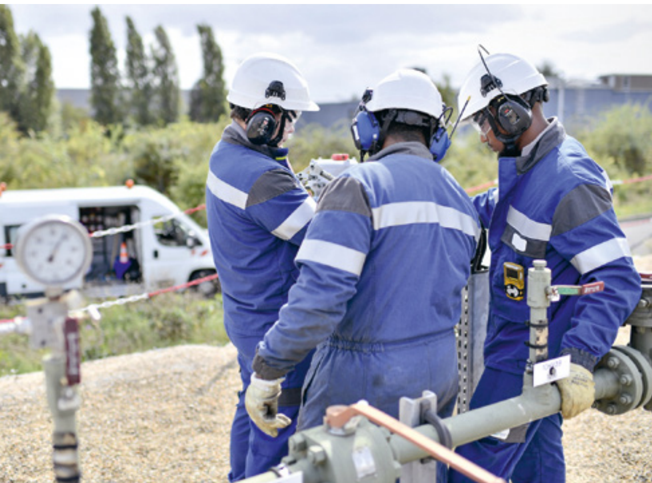
Maintenance on an interconnection station. © GRTgaz/Dunouau Franck
